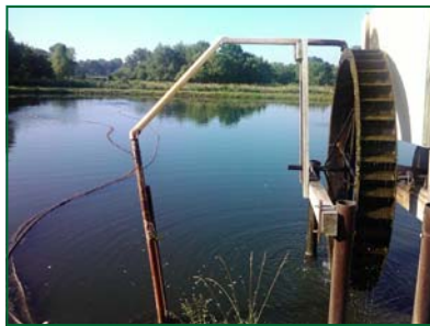
Spring-powered aeration system
