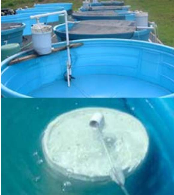
Figure 1. Outdoor green water biofilters at Windward Community College. Top: trickling filter mounted on tank rim. Bottom: submerged filter in tank. Photos by K. McGovern-Hopkins.
